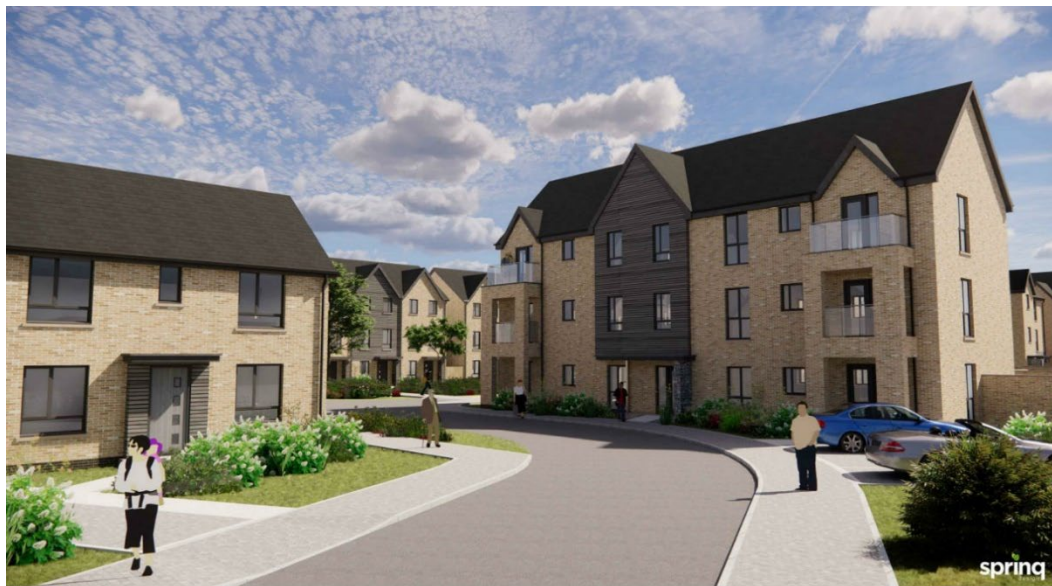
Figure 5: Area One - The Entrance Area
